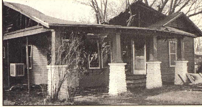
103 Oak Street is lost to early morning fire.
