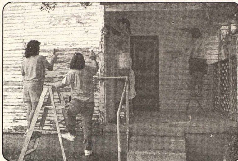
Preparing for new paint at St. Ann's
