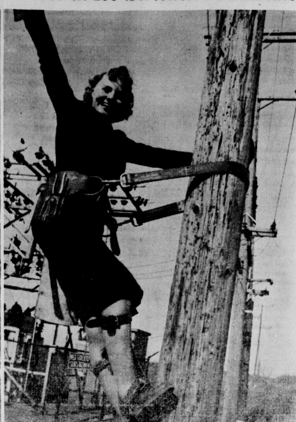
The West Texas Utilities alone had 200 men at work at one time repairing damage wrought by the Panhandle's worst ice and sleet storm. Among volunteers who pleaded for the assignment of "helping out" was a girl, Miss Sarah Smith, WTU cashier at Anson, who said: "I think it's the neighborly thing to do." She proved her willingness by squirming up a 50-foot power line pole.
