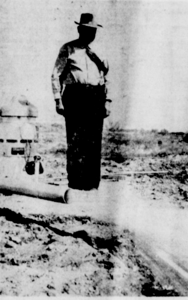
Shown at left is Water Commissioner Edgar C. McGee standing by the new water well that was completed last fall and recently turned into the supply system. Lack of pipe had delayed this well from being put into use. The new well has a capacity of 300-gallons a minute and will be pumped at 200 gallons a minute with continuous pumping as the shallow wells weaken. With all five wells pumping the capacity is expected to be 750 gallons a minute, and additional wells planned for the summer will bring the capacity to 1,000 gallons a minute. Water from the well is 30 per cent softer than from the wells that have been pumped during the winter months. With this well, and the addition of others planned, water supply will be adequate for the swimming pool to open and continue thru the summer months.
