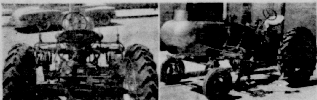
Views of Farmall tractor with a 42 gal. Butane tank.
