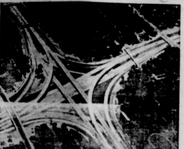
EXPRESSWAYS MEET in this gigantic interchange in Detroit, a key part of the freeway system which could carry some of the Motor City's auto-riding populace to rural safety. Although civil defense studies show that COMPLETE evacuation of large cities after warning of likely attack is not generally feasible under today's warning times, a big start toward more evacuation capacity is being made in urban freeway construction under the new National Interstate Highway program. (Photo courtesy Bureau of Public Roads)
