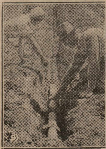
This sub-irrigated row in the garden of Rosa and Rudolph Smaistrla, East Bernard, furnished the family plenty of tomatoes for fall. Such irrigation systems are coming into use all over Texas. They are easy to install and lengthen the garden season.
