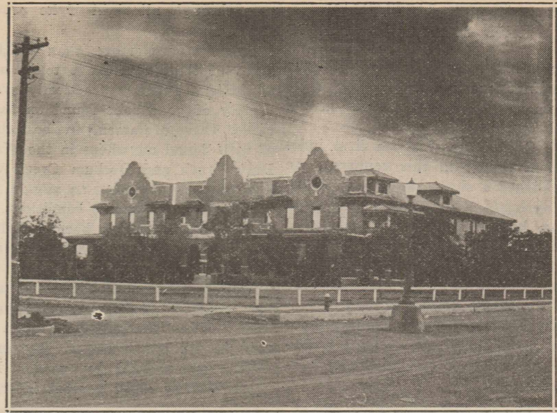
View of the Spur Inn
