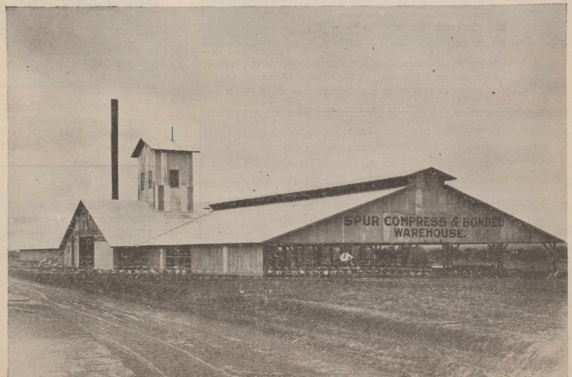
Spur Compress and Bonded Warehouse Recently Completed
