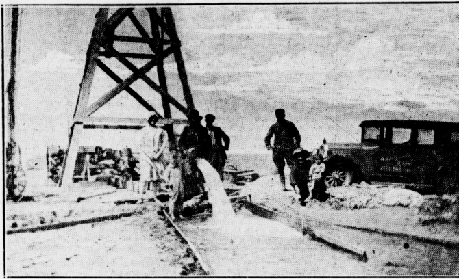
IRRIGATION WELL ON STEEL RANCH SIX MILES SOUTH OF MULESHOE, DELIVERING 1,500 GALLONS PER MINUTE ACCORDING TO TESTS MADE BY DEMPSTER PUMP COMPANY WHO MADE INSTALLATION
