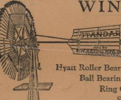
Hyatt Roller Bearings Ball Bearing Turntable Ring Oiling Pitman Self Tightening Wheel
