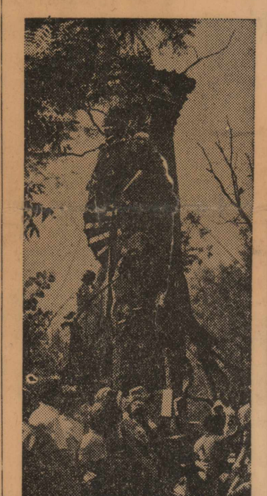
The 44' tall swamp tree slide on Skull Island at Six Flags Over Texas is built around what once was a fire escape at a dormitory at the University of Texas. Guests climb the spiral staircase around the outside of the tree and slide down the long corkscrew-type slide inside.
