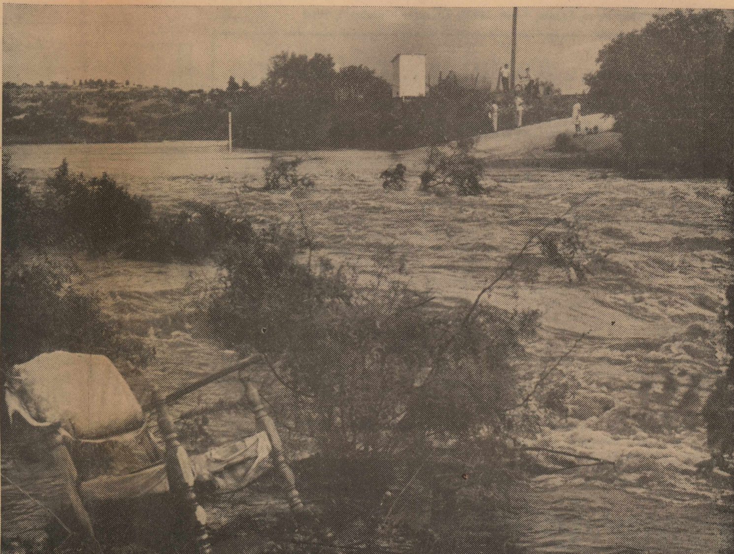
FLOODWATER BOILED AND TUMBLED down Lowrey Draw last Wednesday after four days of heavy rains. The water was being discharged from four flood-prevention dams on the draw.
