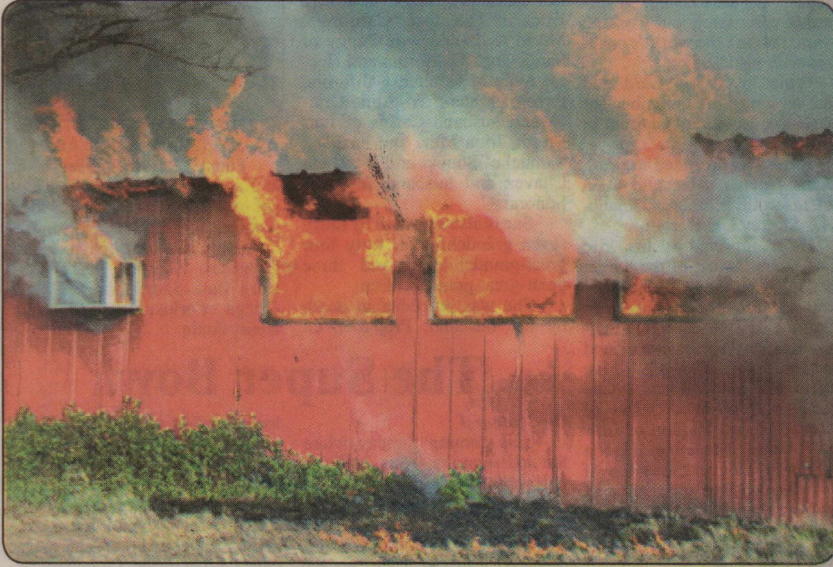
Flames shoot out of the back part of the Hitchin' Post Restaurant. The heat and flames knocked out the windows.
