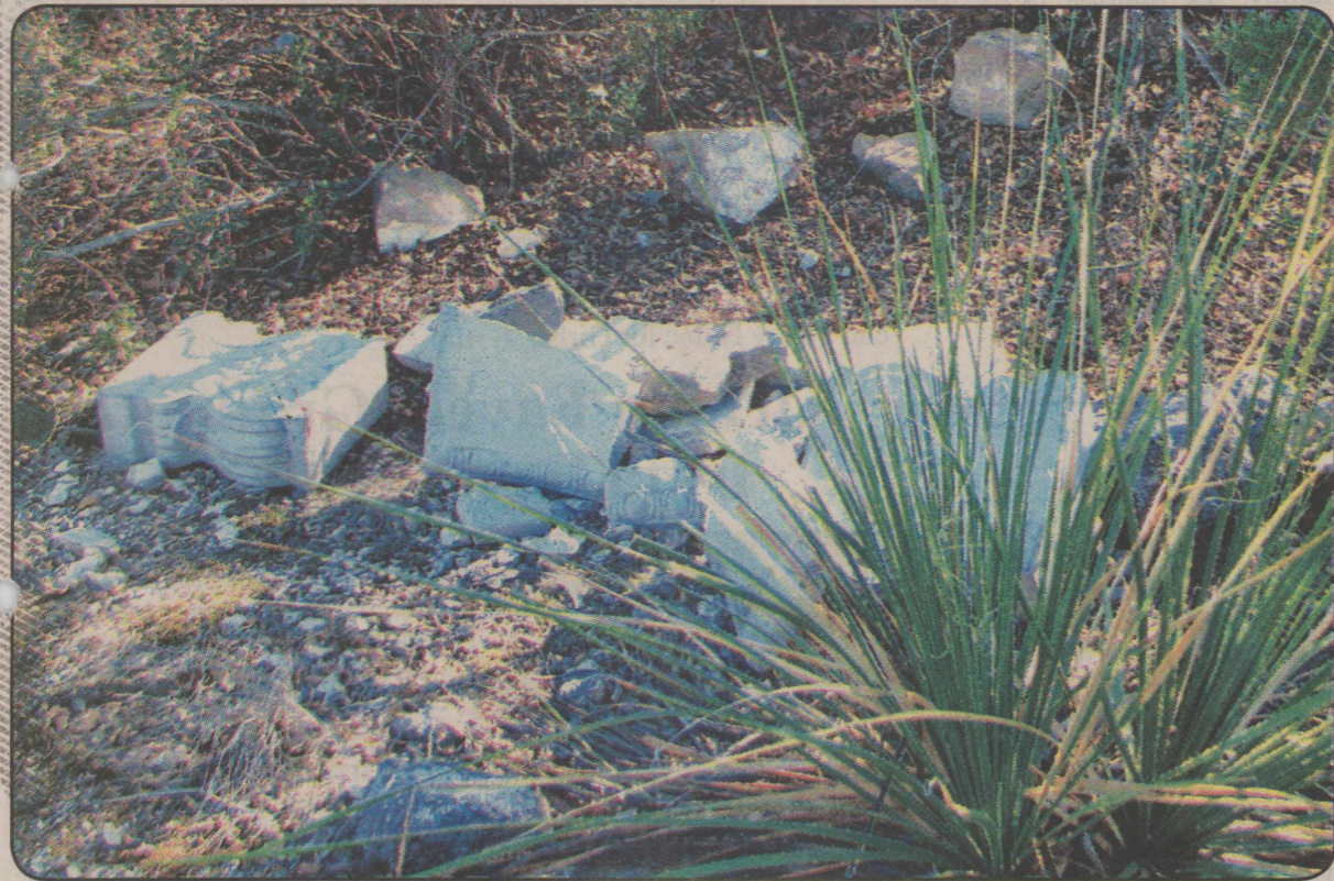
Destroyed concrete bench on Eaton Hill.
