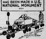
THIS ROAD SURFACE TESTER HAS 18 WHEELS, YET IT IS PULLED BY A SINGLE MAN. EACH WHEEL IS CONNECTED TO RECORDING DEVICES WITHIN THE BOX. THE DEVICE WAS BUILT BY BRITISH ENGINEERS
