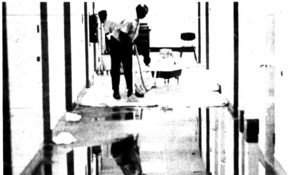
A WATER LINE break this morning at Highland General Hospital flooded three floors of the building. Here one of the hospital's janitors tries to mop up some of the water. The flood occurred when a waterline between two rooms on second floor broke.
