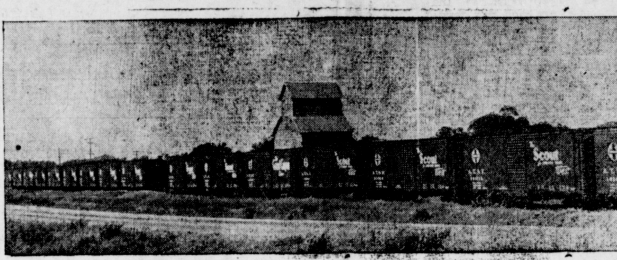
These new Santa Fe Railway box cars stored at a country elevator indicate the preparation being made to handle the bumper 1941 wheat crop. The scene is typical throughout the southwest. Storage facilities for the new crop remain a big problem. Ter-
