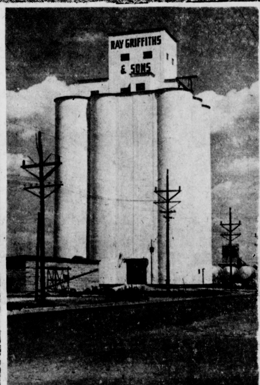
NEW ELEVATOR --- This new elevator recently completed by Ray Griffiths & Sons is one of the most modern in this area. The elevator which has a 300,000 bushel storage capacity, is the tallest structure in Muleshoe and can be seen from several miles while approaching the city from any direction.
