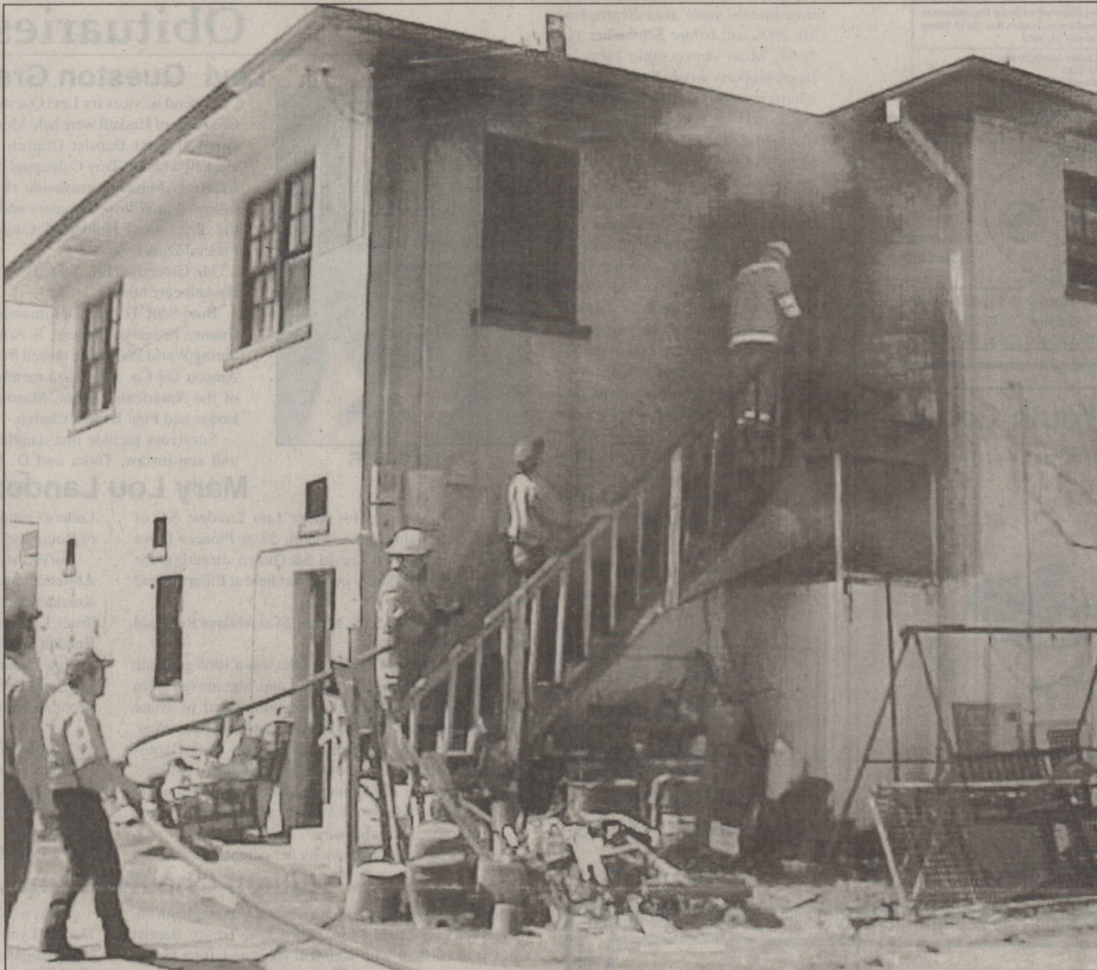
FIRE DAMAGES APARTMENT -A fire at the old Arrowhead Motel location, Wed., Mar. 27 was started by a small charcoal briquet stove on which apartment resident, Jerry Freeman had cooked lunch. Thinking the coals were out he had placed it on the landing
