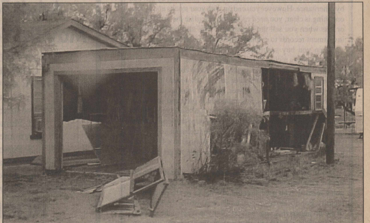
WEEKEND WEATHER HAVOK —The garage of Fred Albright was one of several buildings in the vicinity of Veda's Camp sustaining damage during a storm occurring at approximately 5:00 p.m. Sunday. Twain Mickler reported lots of tree limbs and various items scattered across the field at Veda's Camp. Mickler had measured 1 1/2" of rain by noon on Monday, with more rain still falling.
