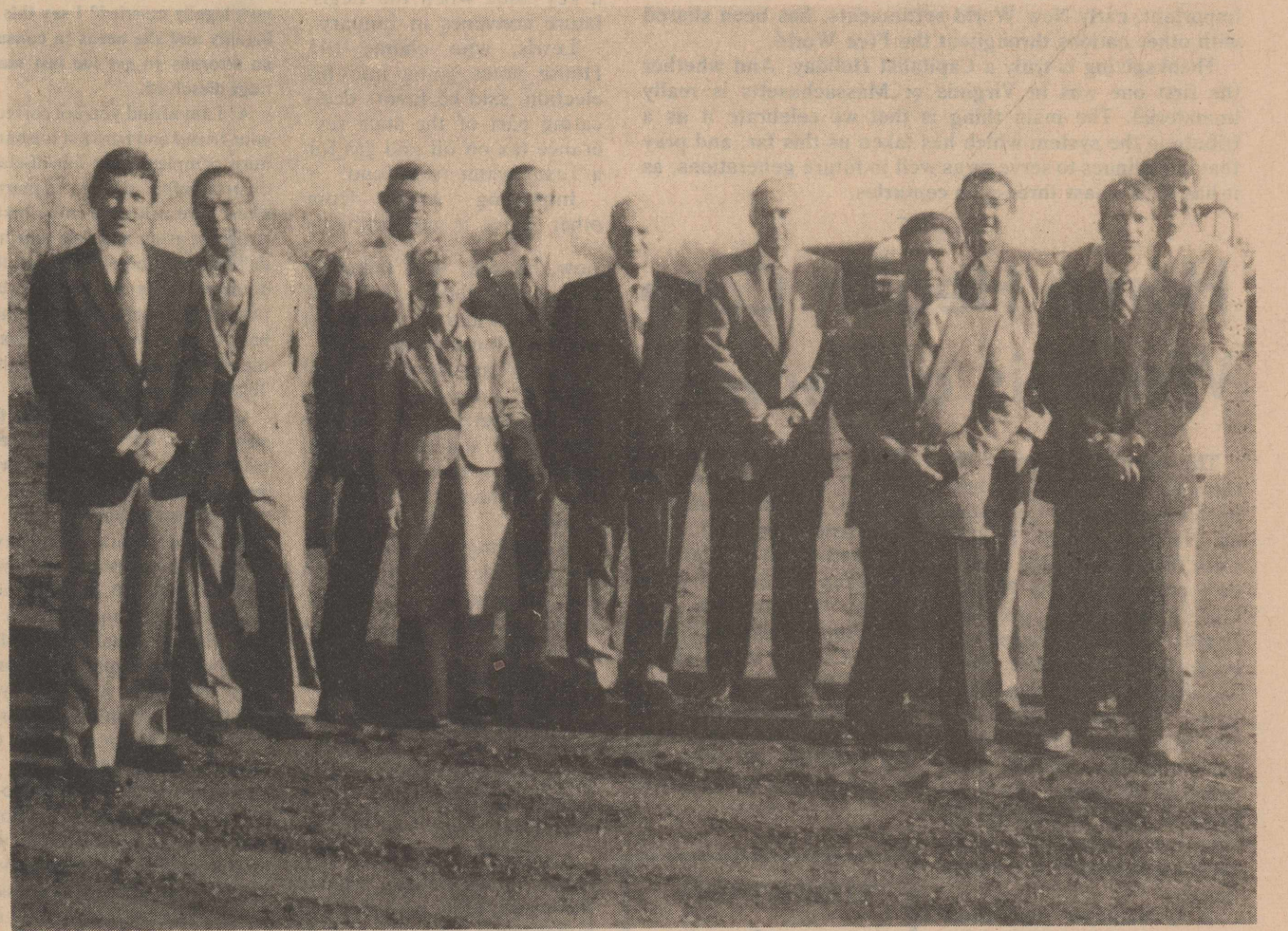
GROUND BREAKING FOR Crockett County National Bank was held Friday at 9:30. Several local residents and the directors of the new bank took part. The bank will be located at Hwy. 163 and First Street. Directors present for the event were Duane Childress, Gene Lilly, Frank McMullan Jr.,
