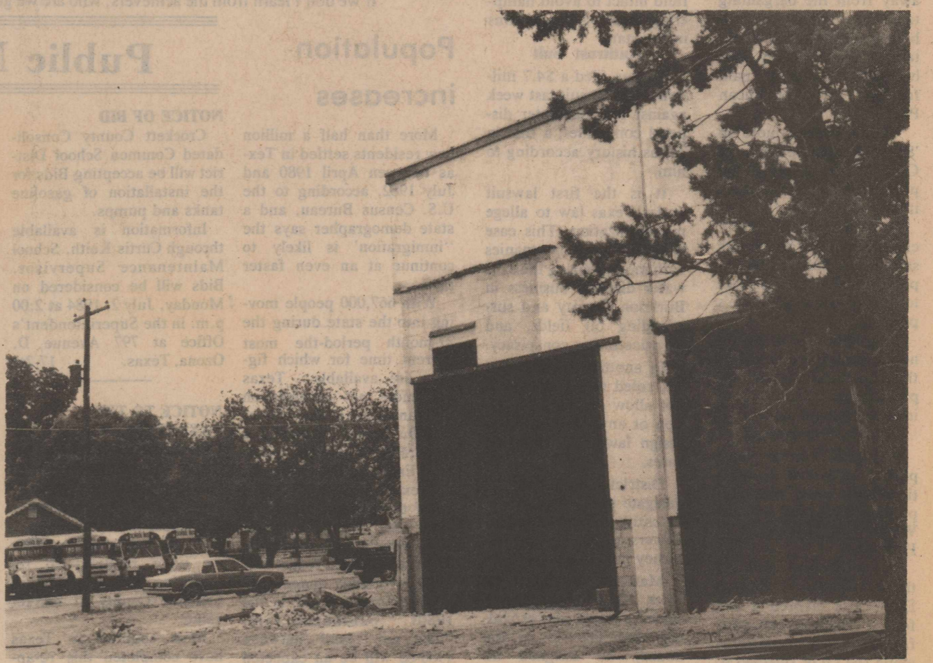
Construction under way
