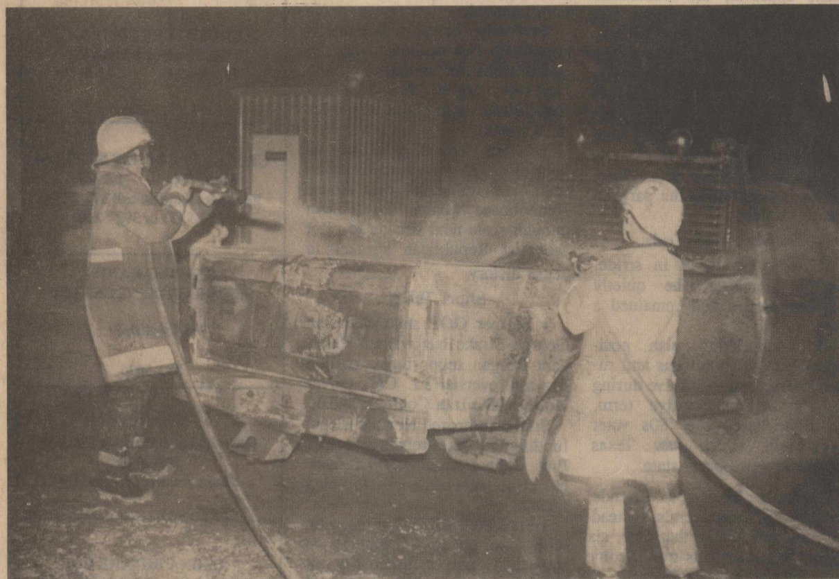
Robert Tambunga and Della Moore put the finishing touches on a fire Monday night at a Hanover Energy gathering station one mile off the Pandale Road. There were no injuries in the fire. Cause has yet to be determined.
