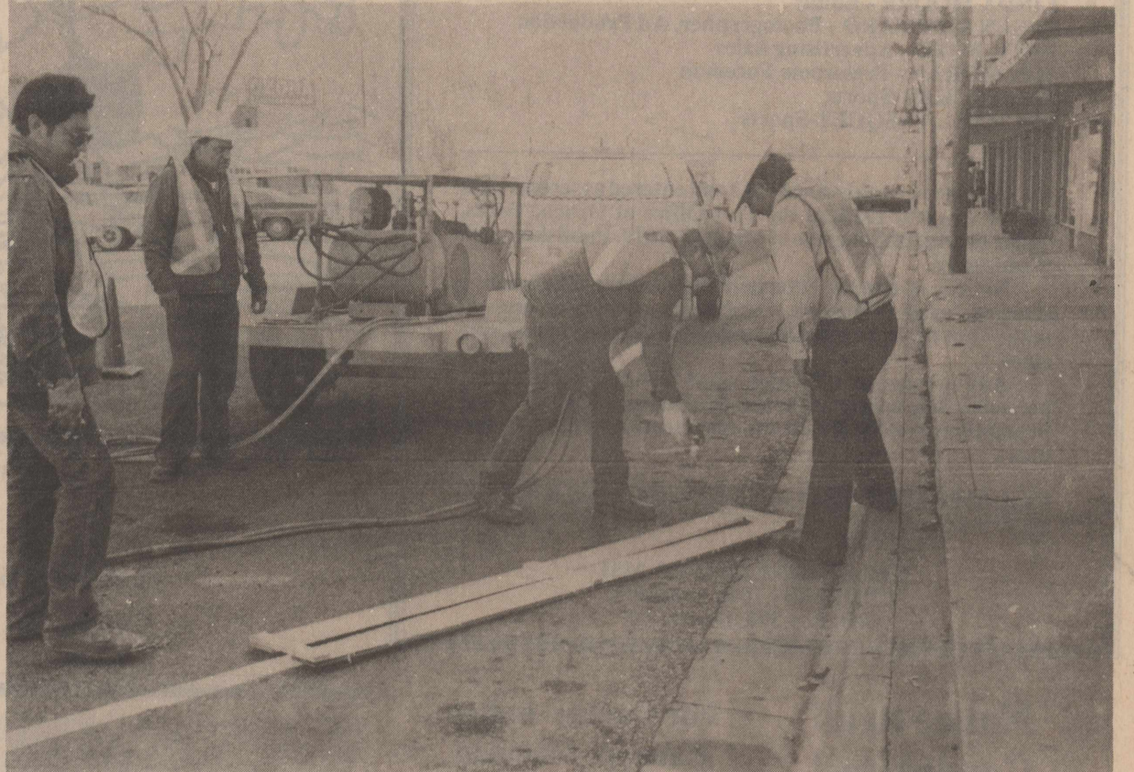
Texas Highway Department employees measured and painted the new parking stripes in the downtown area last week eliminating some parking spaces. The new parking rule was incorporated to insure greater visibility and more room for highway traffic.
