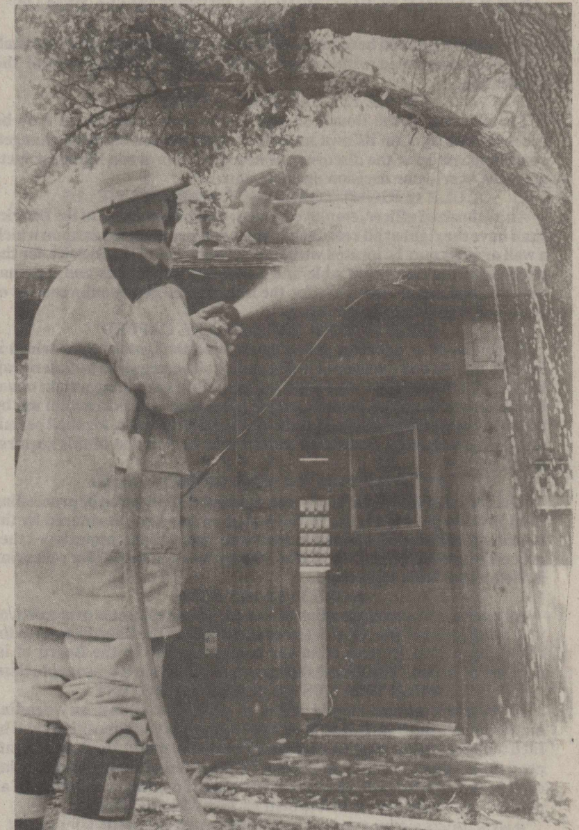
QUICK ACTION prevented a tragedy at a residence on Coates St. last Thursday. Bear Borrego (on roof) lifts a section of the tin so Tommy Miller can douse the flames along the faulty electrical wiring.
