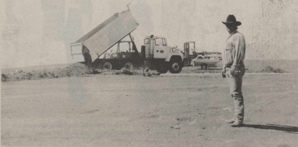
COUNTY ROAD SUPERVISOR EDDIE MOORE inspects the landfill coverup as it nears completion. The job, which began Dec. 1, 1992, has required 27,380 cubic yards of material to cover the landfill.
