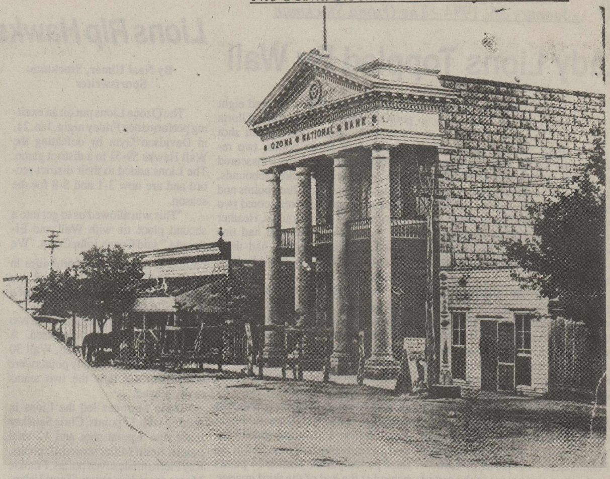
THIS VIEW OF EARLY DAY OZONA is taken from an old post card loaned by Mr. and Mrs. Buddy Moore. Note the wooden frames protecting fledgling trees in front of the bank. The building north of the bank houses the shop of bootmaker Kurt Lange.
