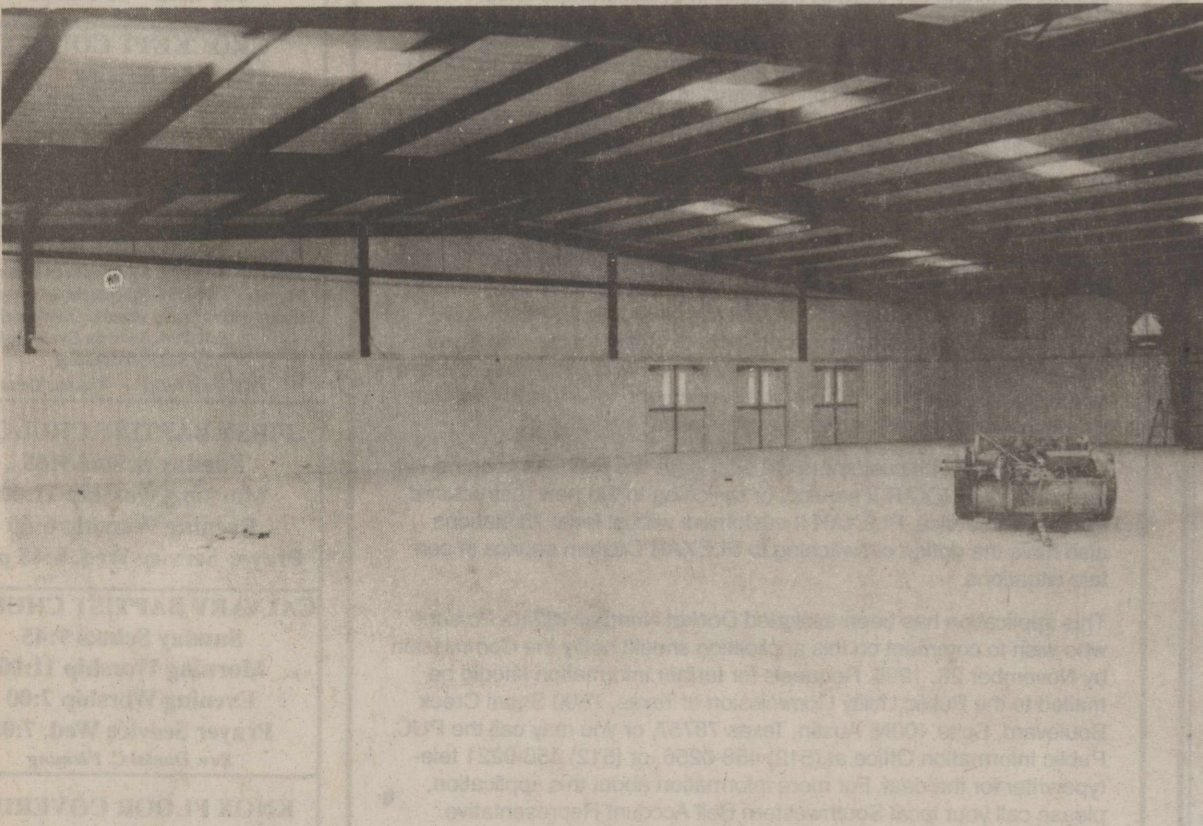
FAIR PARK CONVENTION CENTER - Finishing touches are being put on the building this week. A DeerFest meeting will be held there on Wednesday, Nov. 16, at 7:30 p.m. Anyone interested in helping with 1994 DeerFest is welcome to attend. Photo by Linda Moore
