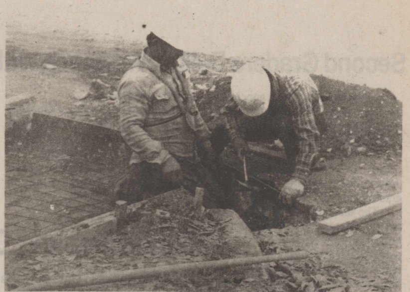
TEXAS DEPARTMENT OF TRANSPORTATION workers are busy building a ramp on 11th Street as part of the requirements to conform with the Americans With Disabilities Act. Once the project is completed, a person in a wheelchair will be able to travel from one edge of Ozona to the other on sidewalks along the state highway. photo by Neal Ulmer
