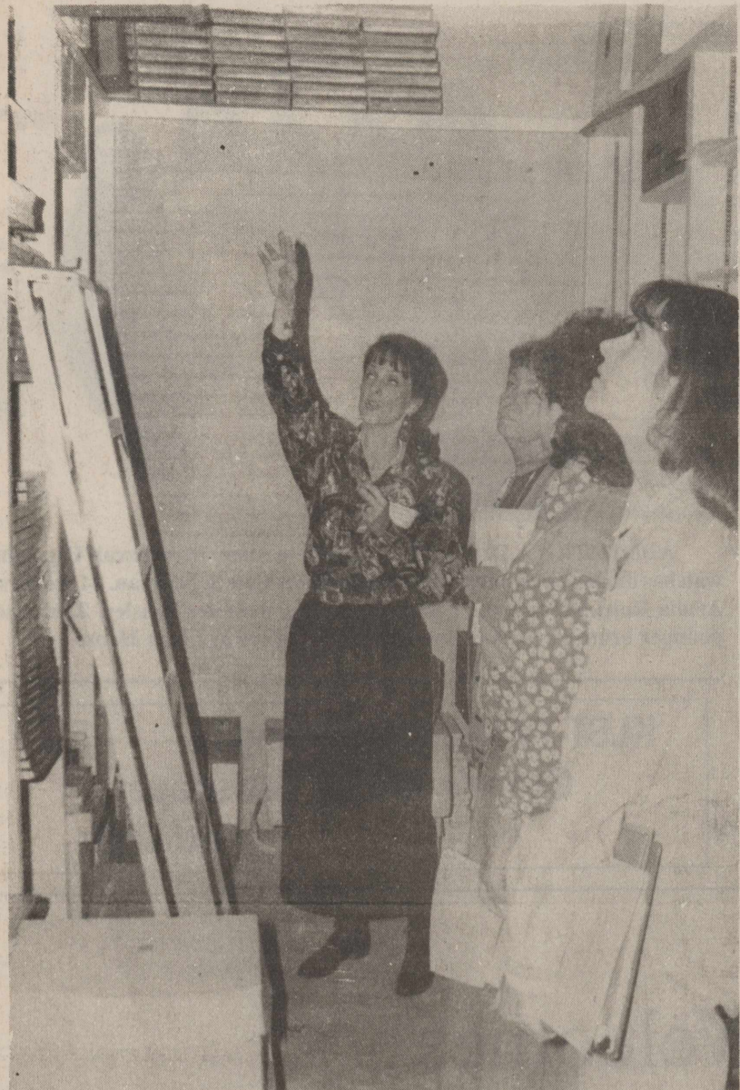
MIDDLE SCHOOL TEACHER MARY ANN DEATON points out deficiencies and needed repairs on the textbook storage room. Other Program and Facility Committee members from back to front are: Shirley Kirby, Charlotte Laughlin and Tammy Bunger who are looking at the damage. photo by Neal Ulmer
