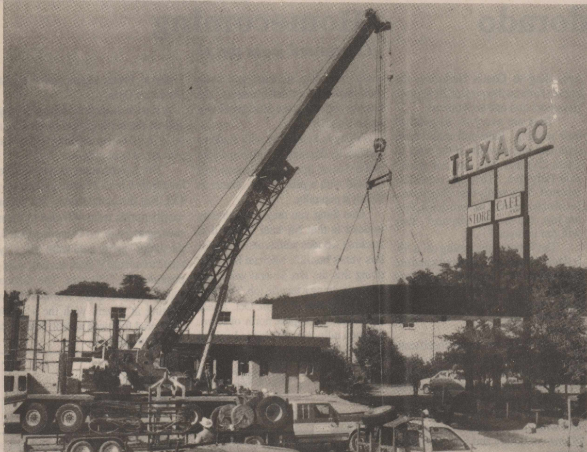
LILLY CONSTRUCTION'S crane lifted the canopy weighing 11,600 pounds over the new fuel pumps at Maness I-10 Texaco last Thursday. Renovations are still continuing but the pumps will be open 24 hours with the use of most major credit cards, ATM or bank cards. Photo by Neal Ulmer
