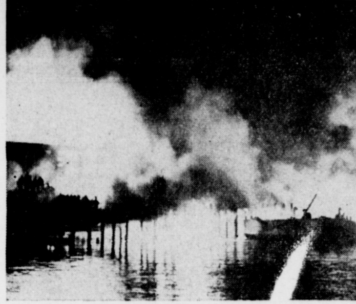
GASOLINE FIRE RAZES PIER — A gasoline barge, shown burning at the right, while pumping fuel into 3 storage tanks at the Tidewater Associated Oil Co. docks in San Francisco, exploded and caused an hour long raging waterfront fire which destroyed two buildings and gutted the pier tanks and barges. Six men are reported missing and there appeared little chance that they survived the fire.
