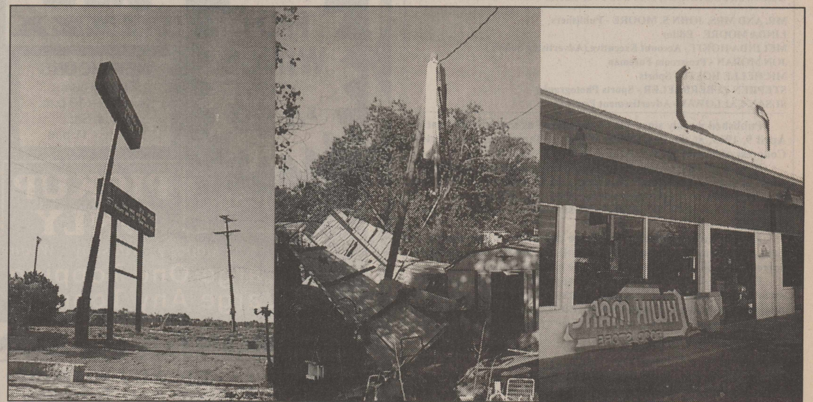
HIGH WINDS IN A THUNDERSTORM MONDAY bent the sign at Comfort Inn (l.) and broke out the sign above the door at Kwik Mart (r.). Half of the second roof was ripped from over the home of Len and Mary Hillman, and part of the metal was draped over the electric lines.
