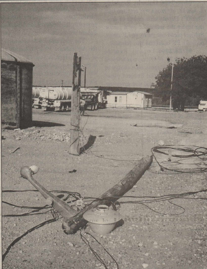
THIS LIGHT POLE was snapped like a twig at the Pool yard north of Ozona during the May 27 storm. Photo by Scotty Moore
