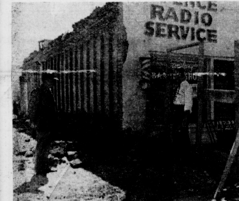
THE WALLS CAME TUMBLIN' DOWN: Charles Moses, barber, and Bob Burkett, real estate, both next door neighbors seem interested in the adobe blocks that made the walls of old buildings on Main Street razed to make a modern new brick building for the Moeller Estate. Adobe walls served a purpose in the early days of the Plains but now are pretty well passe.
