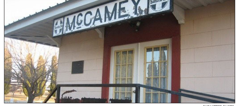
MCCAMEY'S SANTA FE DEPOT will be the site for the Nov. 15 Texas Pecos Trail Region bi-monthly Partners Event, Board Meeting and annual meeting.
