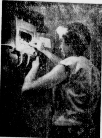
This dilemma is common in too many homes—what she needs is more "housepower". Blowouts due to overloaded wiring can be prevented by the addition of more circuits.
