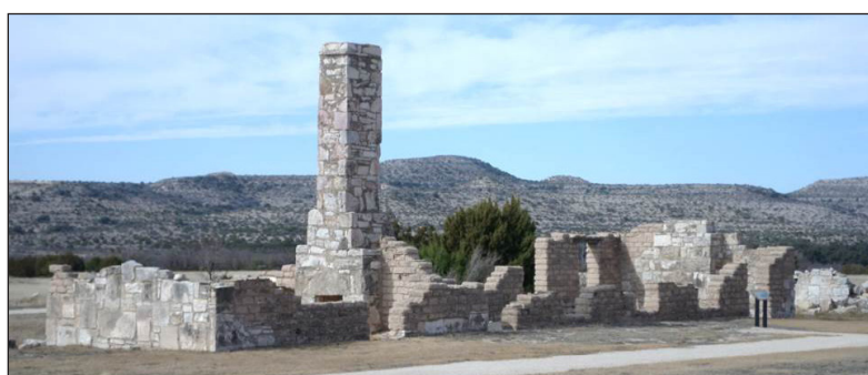
THE RUINS at Fort Lancaster show the remains of the battle that took place there on Dec. 26, 1867.
