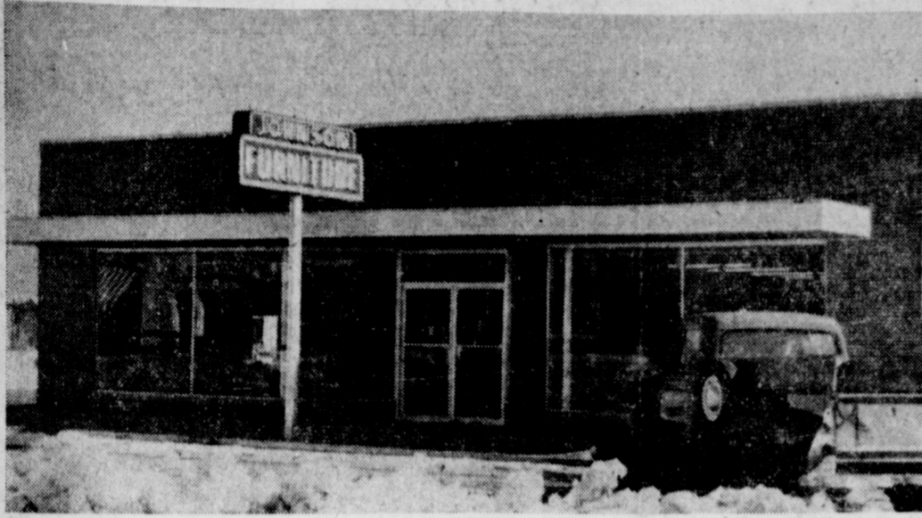
JOHNSON FURNITURE Co. new building located on main street opposite Johnson-Pool. The new store will be the scene of a grand opening sale this week end with representatives of leading furniture companies on hand to demonstrate their products. (Staff Photo)
