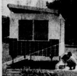
JACKED-UP HALF is lowered onto foundation footings laid earlier. Homes have 680 square feet of living space, sell for \$6,990 each within a 500-mile radius of Leesburg plant. Price includes hauling of six-ton halves and cost of foundation.
