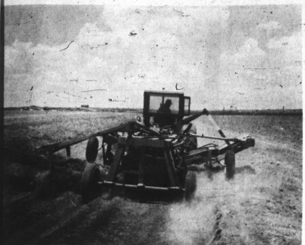
SPECIAL MACHINE — PICTURED ABOVE IS A MALSAM TERRACING MACHINE DOING PARALLEL TERRACES ON THE WALTHALL LITTLEPAGE FARM, TWO MILES SOUTHEAST OF TAHOKA. DOING THE WORK IS LYLE DUGAN, OF BROWNWOOD. LITTLEPAGE IS BUILDING THE TERRACES ON ABOUT 90 ACRES TO CONSERVE WATER AND PREVENT SOIL EROSION, CONSTRUCTING THE TERRACES THROUGH THE GREAT PLAINS CONSERVATION SERVICE. (SCS PHOTO)
