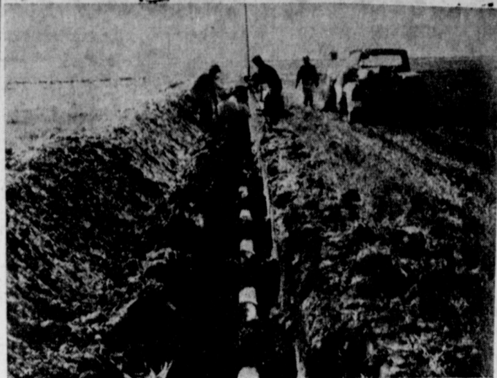
INSTALLATION of cement abestos on Arie Woodfin farm east of Baileyboro for sprinkler system use.
