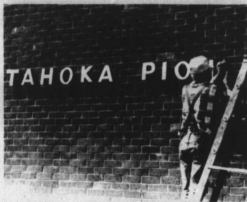
ONE LETTER AT A TIME - Bill Craig of Tahoka places the sign on the newly-bricked wall of the Tahoka Pioneer Museum this week. The letters, made 14 years ago by Craig, are made of scrap metal, including "pieces of old John Deere tractors and such." Craig said the building housing the museum on Lockwood Street was formerly a gas station and car dealership, and the museum was opened 14 years ago.
