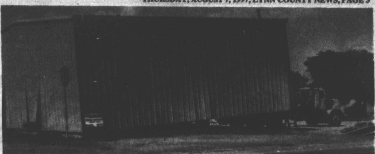
BUS BARN MOVES ACROSS THE STREET - Tahoka L.S.D.'s tan bus barn was moved across the street by the Home Ec building last week, in preparation for erecting a new ag shop/classroom building in its place, on the corner of N. 2nd and Ave. P. Tim Walker Construction Co. is building the new facility in a style similar to Tahoka's new Life Enrichment Center. (LCN PHOTO)
