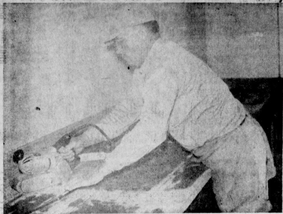
HITTING THE HIGH SPOTS — W. O. Browder, maintenance man in the Mule-shoe schools, is shown above as he sands down one of the work tables in the chemistry laboratory. The tables will be covered with fomica for a smooth working surface.
