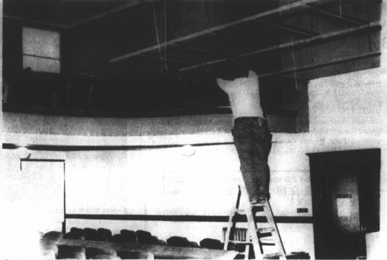
CEILING REPAIR - Andy Dunlap completed installation of a new ceiling and recessed lighting in the Lynn County Courtroom this week, after a freakish lightning strike destroyed the ceiling recently. The old balcony and goldleaf trim high on the old walls are visible while Dunlap works on the dropped ceiling. The balcony, however, was once again hidden when the new ceiling work was completed (photo at left). The repairs give a more modern look, and better lighting, to the district courtroom. (LCN PHOTOS)
