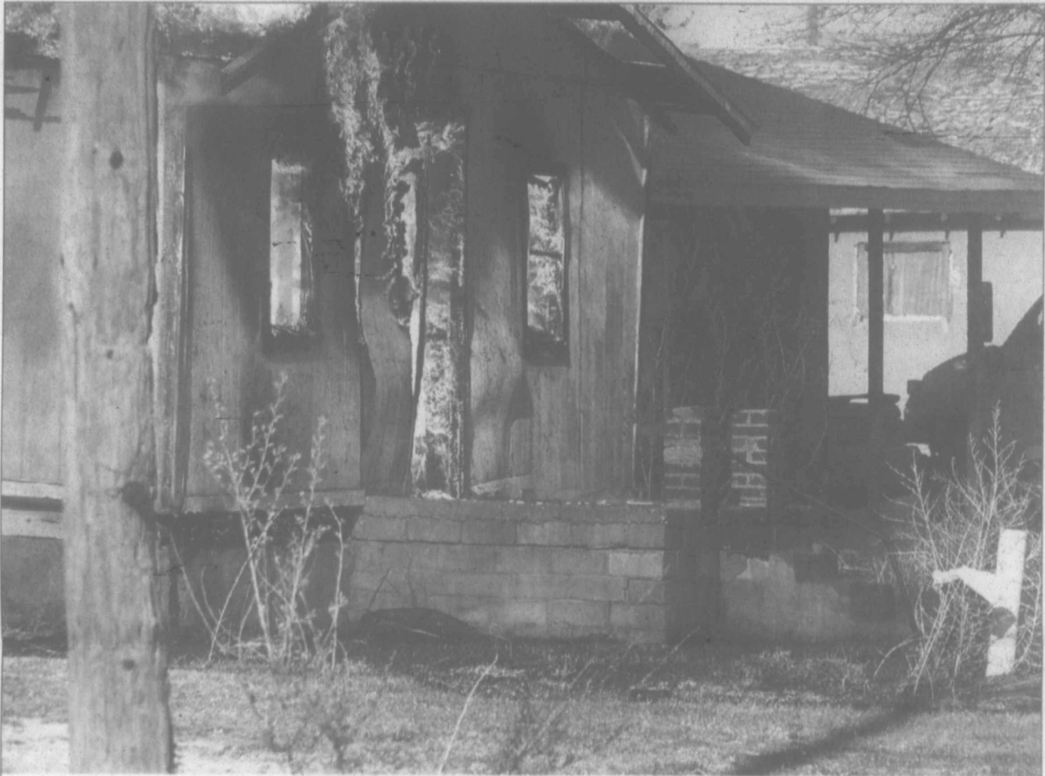
Big blaze ... Fire consumed this abandoned house in the 1200 block of North 5th Street Monday evening, as Tahoka Volunteer Fire Department responded. Thankfully the winds were light that evening, and firemen were able to contain the fire to the abandoned house, although some damage to windows was reported on the Anthony Gonzales house next door.
