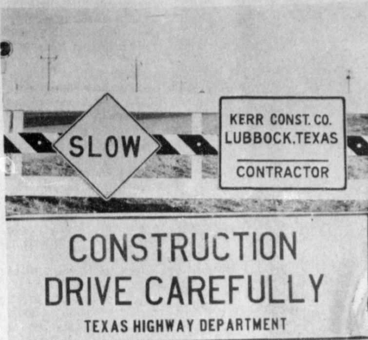
SIGNS GO UP —The first signs of work which has begun on the Highway 84 are the signs of construction and warning signs along with flashing lights. The signs went up shortly after Kerr Construction received work order this work.
