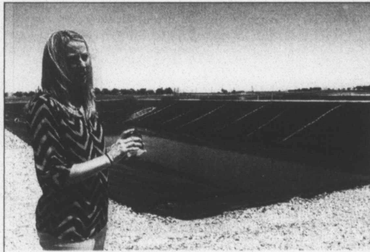
New wastewater plant ... Kori Welch, an engineer from Parkhill Smith & Cooper, Inc., is pictured in front of the facultative lagoon at the new wastewater treatment plant in Wilson, as she explains the treatment process. (LCN PHOTO by Juanell Jones)
