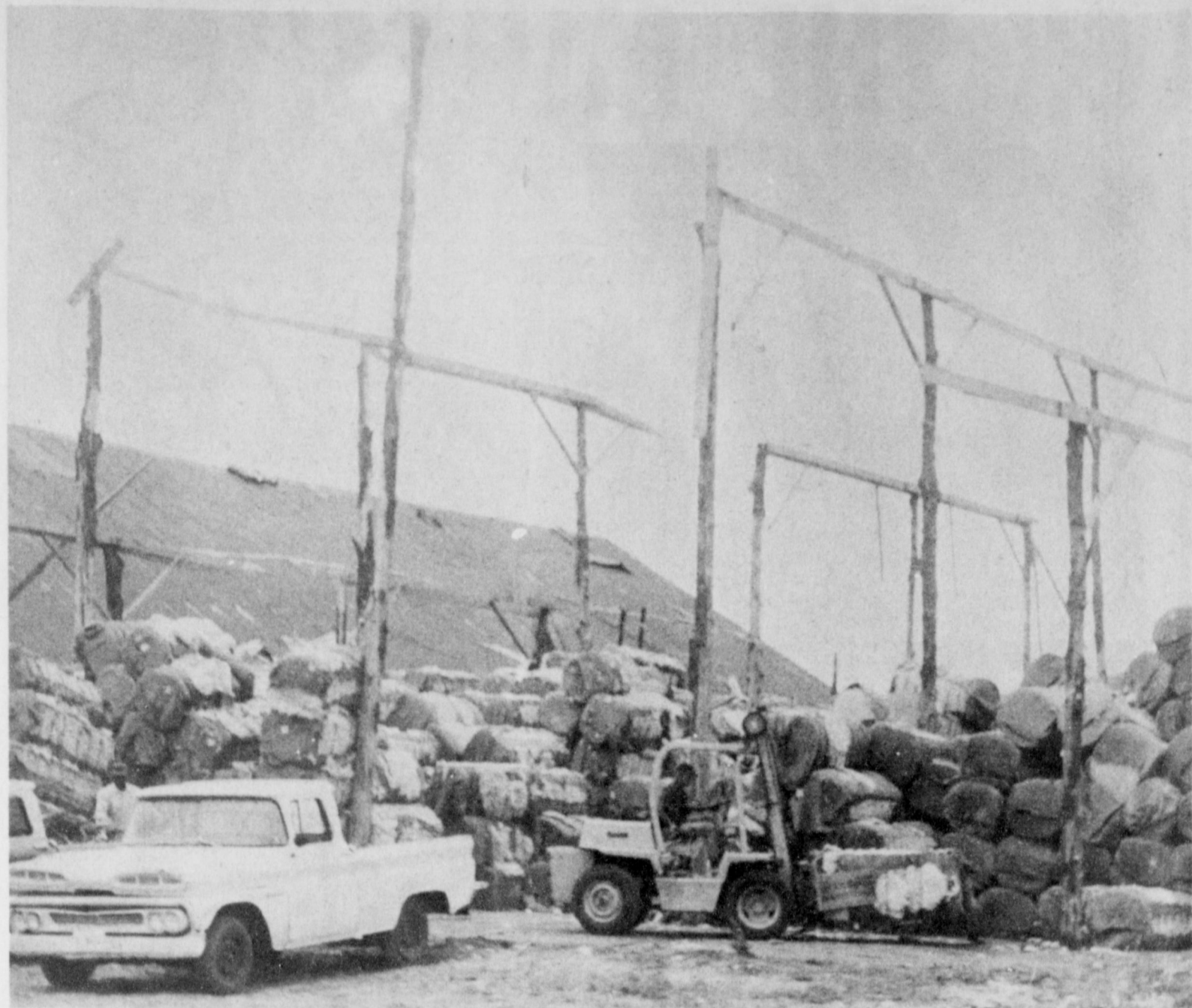
SALVAGE OPERATION--Workmen are cleaning up the wreckage of the Central Compress warehouses, filled with baled cotton which was blown away as a twister dipped to the ground during Sunday night's storm there. The cotton, not damaged is being moved to other storage buildings from beneath some of the building framework left standing.
